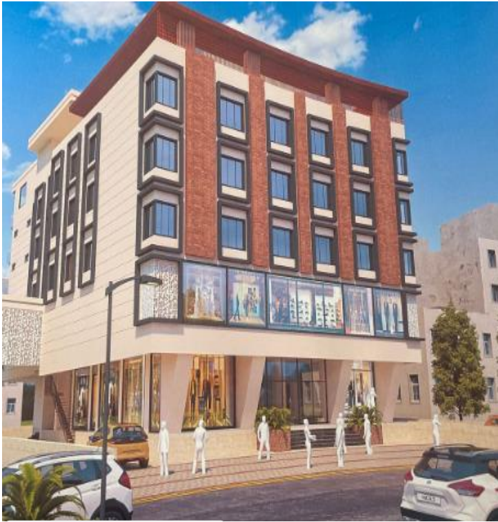
The hotel frontage
